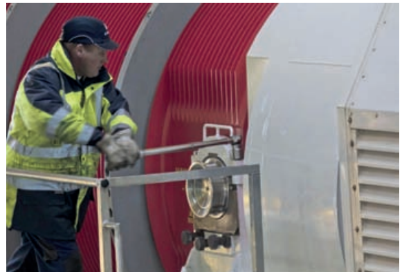
Bolting the CASTOR HAW 28M package onto its chassis
